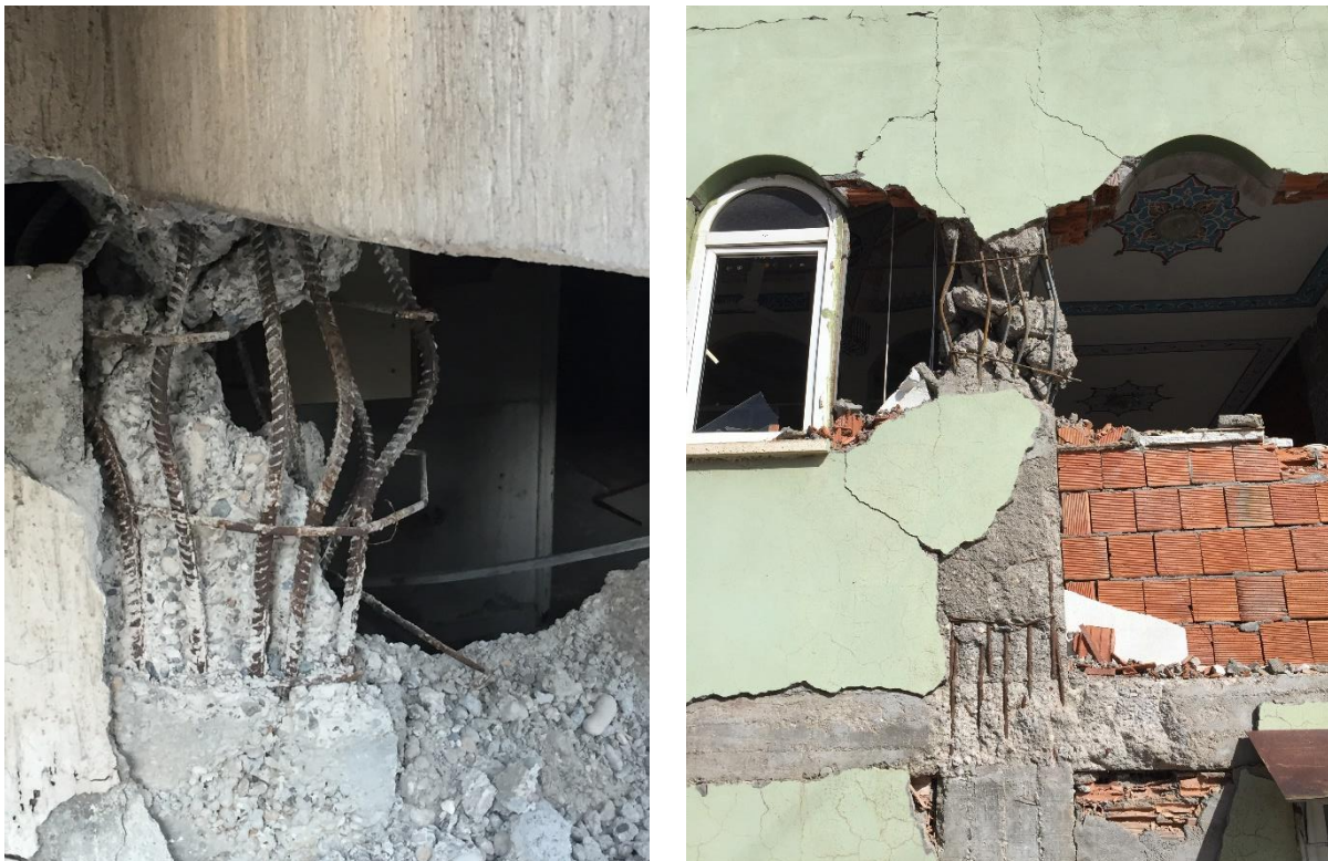
Figure 1. Buckling damage
