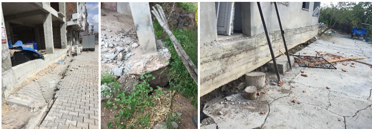
Figure 10. Soil/foundation damage
